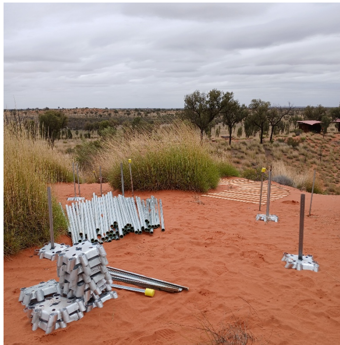
Figure 15 Construction site of lookout platform with view to Camp 2, 13/02/2026
