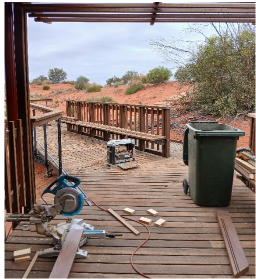
Figure 19 Construction works at Big Wiltja at Camp 3, 13/02/2026
