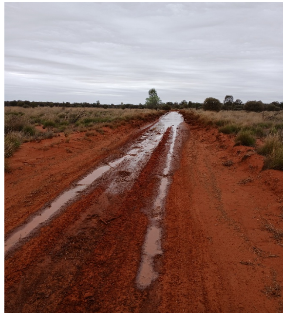
Figure 23 Access Road to Camp 3, showing large water puddle and vehicle tracks, 13/02/2026
