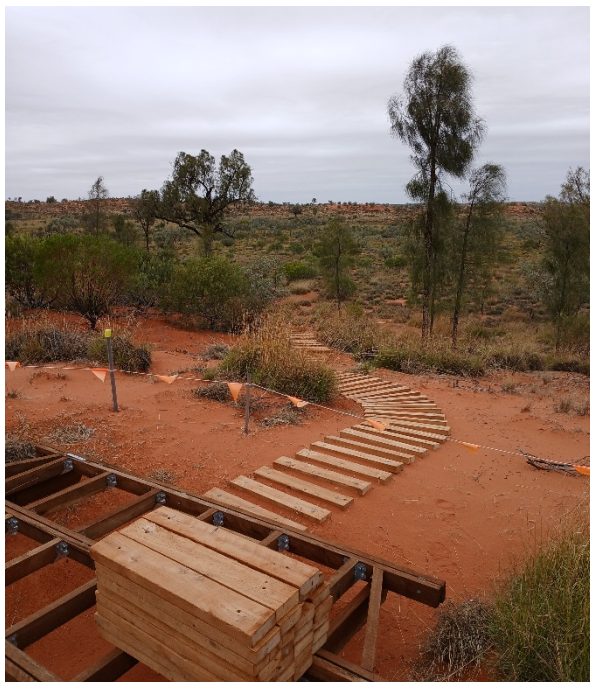
Figure 8 Construction site of Camp 1, showing dune top lookout platform and chain linked timber walk into Camp 1, 13/02/2026
