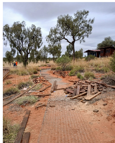
Figure 13 Piles of construction material along access walk at Camp 2, 13/02/2026
