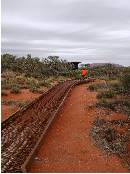
Figure 16 Elevated steel mesh walk from service shed into Camp 3; flagging fence and steel mesh mats have been removed, 13/02/2026
