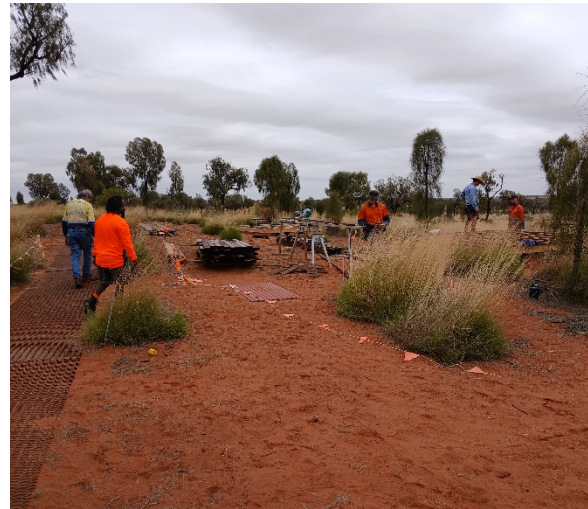
Figure 11 Construction works around sleeping platforms at Camp 2, showing degraded flagging fence, 13/02/2026
